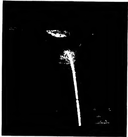
FIGURE 131. "Shotting," in the Byers-Aston process for making wrought iron, by pouring liquid iron into liquid slag. (Courtesy A. M. Byers Co.)
